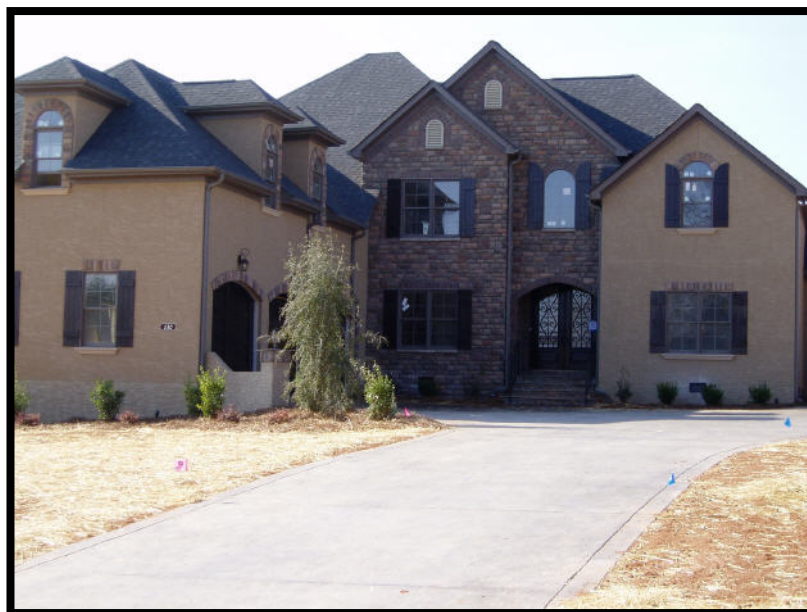
Finished Bellevue by Builder located in Walden Ridge
