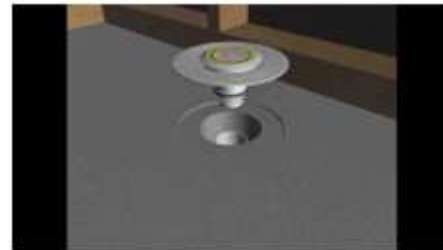
Recess concrete or AC sheet using a grinding wheel so that the puddle flange sits flat with the floor. Glue screw the puddle flange into position. Refer to manufacturers directions
