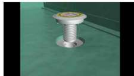
After the waterproofing is complete re-install puddle flange cap to prevent any building debris from entering plumbing untill ready to bed and tile
