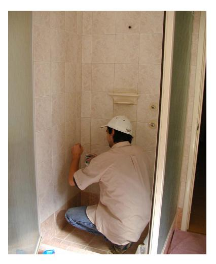
The above shower had cracked grout around the base and hairline cracks in the grout at knee level on both walls. All cracked & suspect grout was removed and replaced with grout mixed with Grout Bond & Seal 4. The hairline cracks were sealed with a slurry of grout and Grout Bond & Seal 4. The rest of the grout in the walls & floor were sealed with Grout Seal 16.
