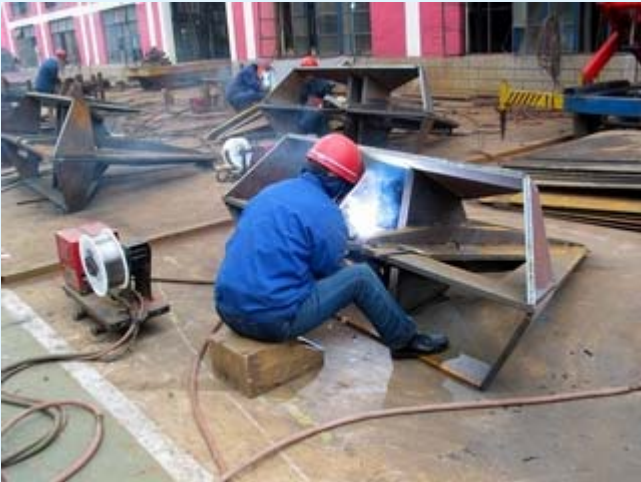
Delta Anchor Fluke - Welding
