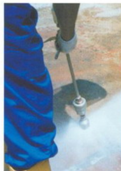
Wide Blasting area with RJ 3000 System
