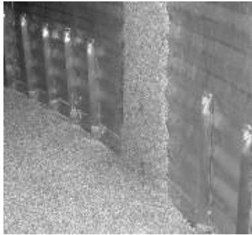
An Airways® Door Kit was not used in this bin. Notice the spoilage in the area not covered by Airways®
