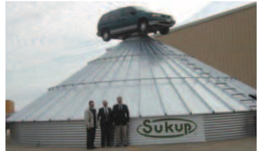
The strength of Sukup roofs starts with high-strength steel. Each sheet is rigidized every 4" to increase the stiffness of the panels, making them easier to handle.
