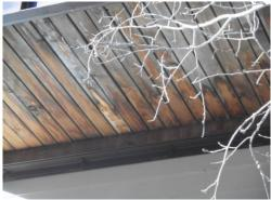
**Description:** 2<sup>nd</sup> floor unit balconies are constructed with a cantilevered metal frame with 4x4 wooden supports and 2" x 6" deck floor boards.
