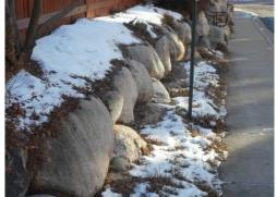
**Description:** Estimated 910 linear feet of stacked boulder retaining walls at a range of 3 to 7 feet in height.
