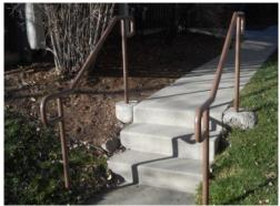
**Description:** Estimated 530 linear feet of metal railings embedded into the concrete surface, adjacent to the concrete stairs.
