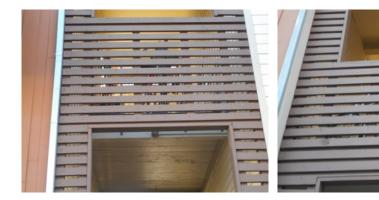
**Description:** Estimated total of 8,875 square feet of 2" x 4" boards that frame within the opening of breezeway common areas that vary in horizontal and vertical lengths.
