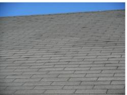
**Description:** Estimated total of 656 squares of laminated asphalt shingles over a membrane. The carports have not been included but are estimated to cost \$60-65k.
