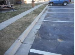
**Description:** Estimated 2,070 linear feet of 6 inch tall, spill and catch barrier concrete curbs with 1- and 2-foot wide gutters.
