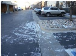
**Description:** Estimated 2,520 square feet of 3-foot wide, reinforced concrete pan, sloped to convey stormwater runoff.
