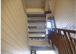
**Description:** Typical breezeway stairs consist of structural wood framing, 2" x 6" wood floor board landing area, attached 3.5 feet high guard railing, attached drainable metal treads, and a detached handrail (single bar) anchored to the condo building.
