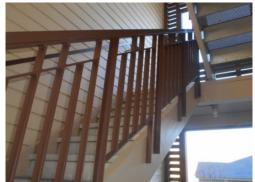
**Description:** 2<sup>nd</sup> floor breezeway entries are constructed with 2" x 10" deck joists, attached to the condo buildings, spanned with 2" x 6" deck floor boards and 3.5 feet high guard rail protection around the open drop-offs.
