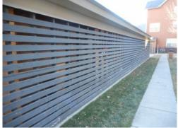
**Description:** Five garage buildings that incorporate cementitious lap siding, hard board products installed as fascia, soffit, paneling, and window and door trim, and wood features at varying lengths of horizontal and vertical 2" x 4" boards. The roofing material used on the garages is laminated asphalt shingles. We were informed by the Association the garages are not their responsibility. Garage improvements are funded seperatley as not all condo owners have a garage space.
