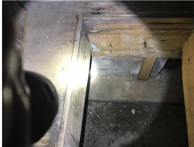
View of crawlspace and footer in Building C-unit #19
