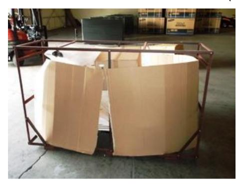
STEP 2: REMOVE METAL FRAME FROM CRATE (USE CAUTION AROUND SHARP METAL EDGES)
