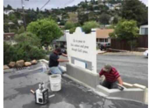
Jose smoothing the concrete base and Nieves applying a masonry finish coat prior to painting.
