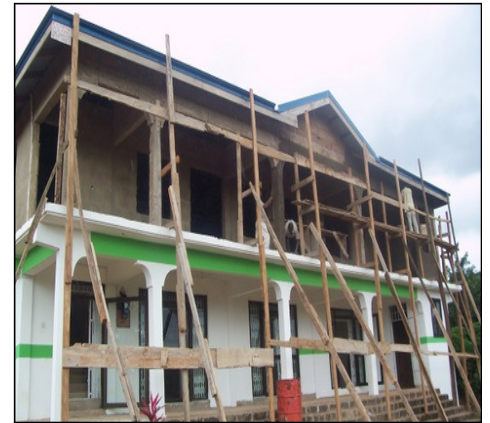
We are getting ready to finish out this phase
