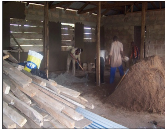
Preparing to plaster the second floor
