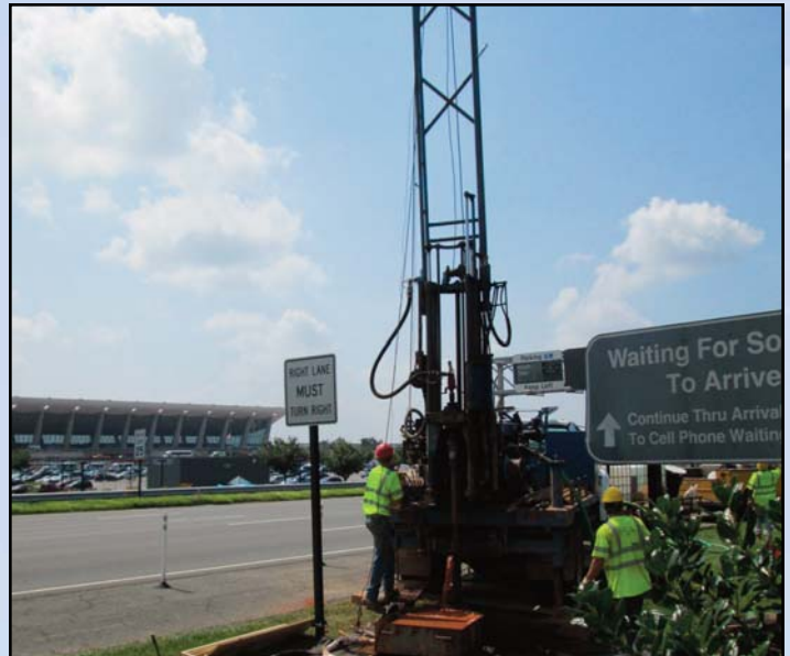
AT THE AIRPORT: Geotech boring samples for future aerial pier location at Saarinen Circle at Dulles International Airport. Photo by Scott Evans, Dulles Corridor Metrorail Project
