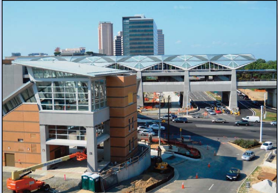
ALONG ROUTE 123 AT TYSONS CORNER CENTER: The canopy of the Tysons Corner Station on the northwest side of Route 123 shines in the sun. At left foreground, the pedestrian pavilion that leads to a bridge for rail users to cross Route 123 to enter the station. In the background is Tysons Galleria and the Ritz Carlton. Photo by Stephen Barna, Dulles Corridor Metrorail Project
